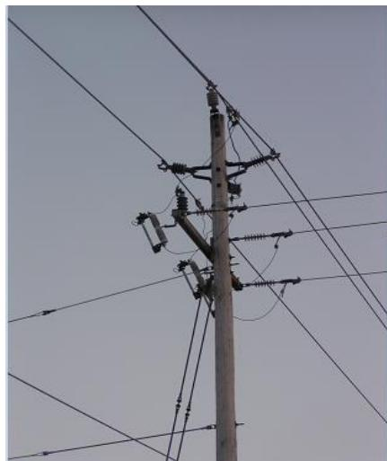
**Figure 3-1, Typical Fused Tap Framing**
