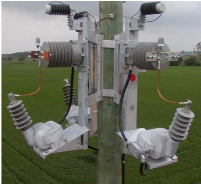
**Figure 6-1, Typical Primary Metering Unit**
