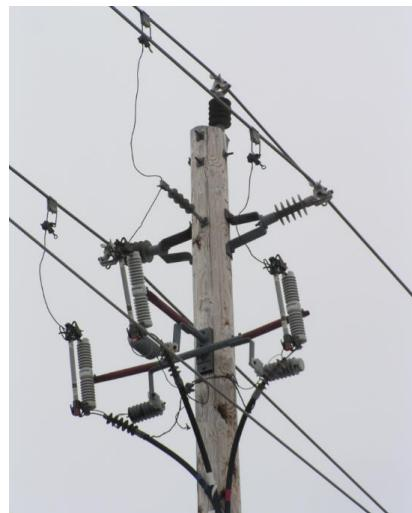
**Figure 3-2, Typical Fused Riser Framing**
