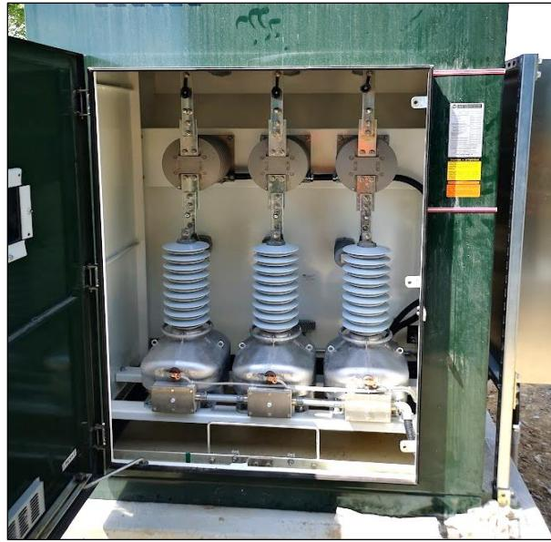
**Figure 3-7, Typical Primary Metering Unit**
