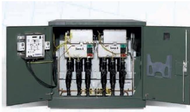
**Figure 3-5, View of Switchgear Interrupter Switch Compartments**
